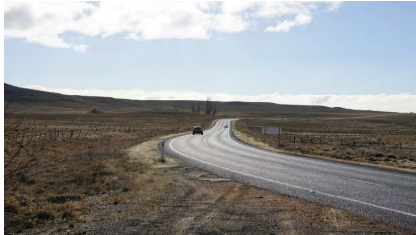
Figure 3.9: Looking north towards Cooma from the proposed access
