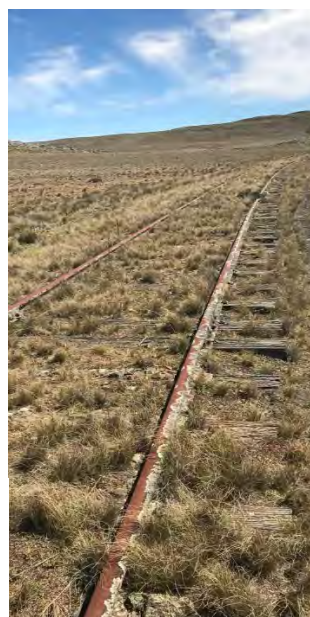
Figure 3.9: Detail of disused railway line across property
